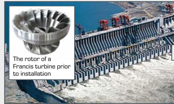
The Three Gorges Dam in China on the Yangtze River uses Voith Siemens Hydro Power Generation turbines.
