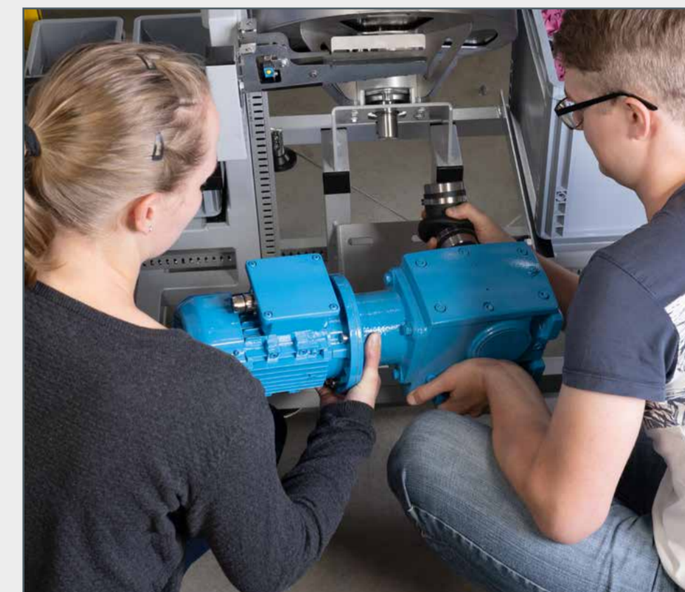
drive train is lifted out, cardan joint is loosened
