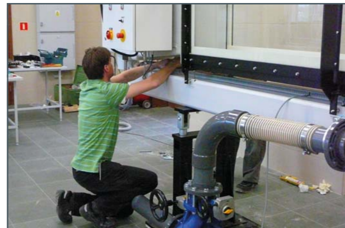
Last but not least is work on the wiring (left). Then the water tank is aligned and connected to the pipeline system (right).
